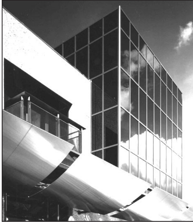
Fig. 5. PV curtain wall “cube” at APS facility in Fairfield, California. The BIPV system includes amorphous silicon PV modules in standard curtain wall framing. The framing is at a 76cm x 152cm (2.5' x 5') spacing. Ten of the glazing units at the left center of the cube are tinted vision glass.
