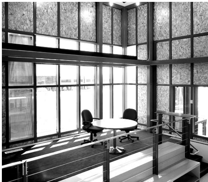
Fig. 6. Interior view of PV curtain wall at APS. For comparison, two of the PV panels to the left of the vision area are left unsealed, showing the relative transparency of the modules.
