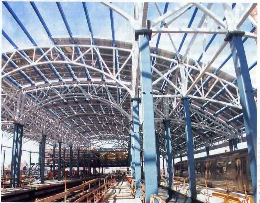
The Stillwell Avenue subway station, in the New York City borough of Brooklyn, features an arched roof integrating 2,730 photovoltaic panels that will generate 250,000 kWh of electricity annually. The roof is supported by arch trusses that span from one platform to the next in neo-Victorian fashion.
