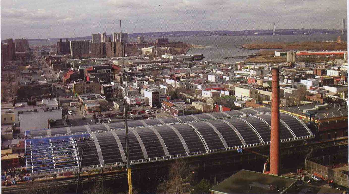
This spring, the Metropolitan Transportation Authority unveiled a 210-kW installation on the roof of its newly renovated Stillwell Avenue subway station.
