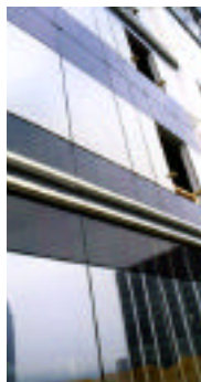
stalled in curtainwall
