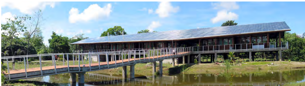
SMITHSONIAN TROPICAL RESEARCH FACILITY, BOCAS DEL TORO, PANAMA, 2005 DESIGNED AS A ZERO ENERGY/ZERO WATER BUILDING, IN A DEMANDING TROPICAL CLIMATE
