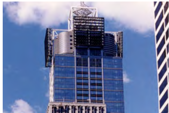
Custom sized BIPV modules developed under a K+C NYSERDA contract were used in Four Times Square
