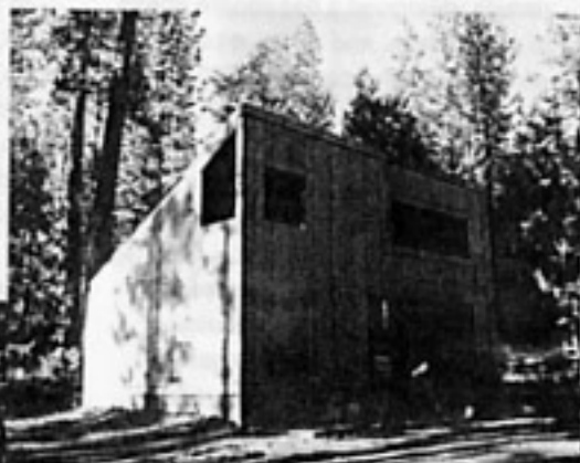
At end of day, shell of Wright house is complete.
