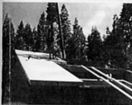
Caulk, adhesive, and long panel screws secure roof panels to wood beams and steel framing.
