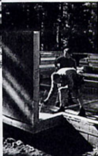
Workers prepare wall-to-floor connections with sealant and adhesives.
