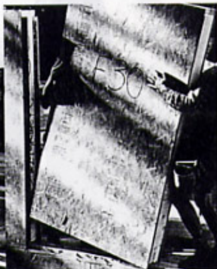
Double-spline joint and bottom plate anchor standard 4'x8' SIP panel into place.
