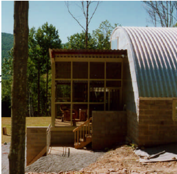
screened porch from north
