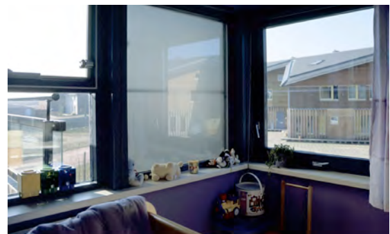
Solarium interior showing semitransparent PV glazing (between glass windows.)
